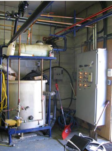
As you can see in the above pictures the condenser water tank is located directly above the trench where the steem brine mains feed the arena floor and picture on the right also displays the water overflow connection from the tank that drains into the trench. Combinatin of pipe age and wet environment in the trench had contributed to the resting and deteriorating of the steel brine mains in question. This also applied to the mains that were feeding the curling rink twards the zamboin room.
