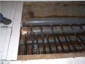
Although the above photos are not taken from the Northern Light Recreation header trench, I just wanted to use them as illustration of how the headers get connected to the pipes inbeded in the concrete floor. As you can see there are lots of pipes the are buried in the concrete (256 to be exact on the cooling floor) and (anywhere from 56 to 86 on the warm floor) depending on the pipe spacing.
